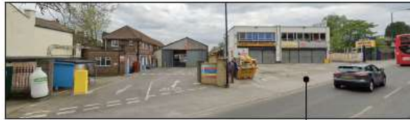
VIEW A - VIEW FROM GAP ROAD SHOWING FRONT ENTRANCE, SERVICE YARD, DROPPED KERB AND NEIGHBOURING BUILDINGS
