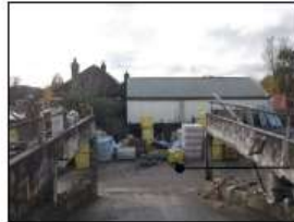
VIEW G - SHOWING RAMP AT REAR - VIEW FROM BACK OF SITE.
