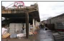
VIEW E - SHOWING ACCESS DOWN RIGHT HAND SIDE OF SITE
