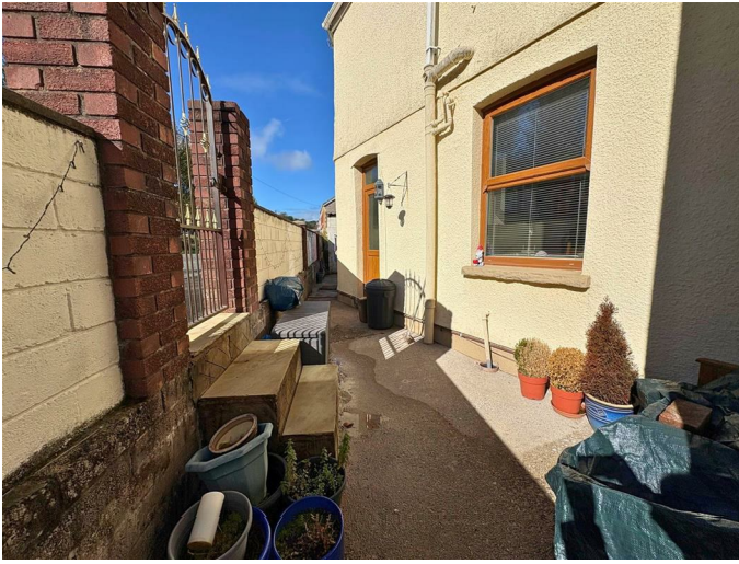
Courtyards laid to concrete with storage shed to the rear, wrought iron pedestrian gate to the side providing side access, bordered with block walls.
