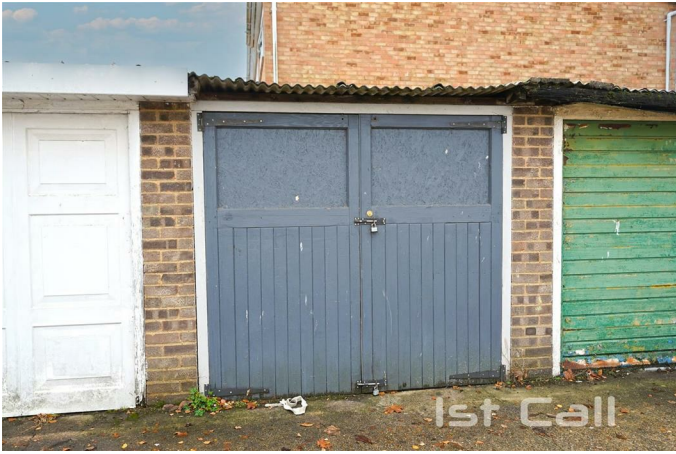
In block with twin timber doors...
