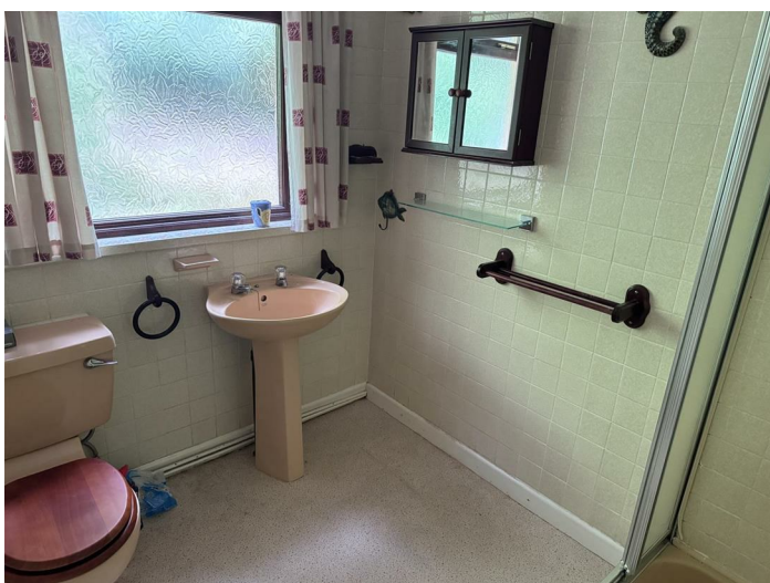
Central heating radiator. Low-level WC, wash basin and shower cubicle with electric shower unit
