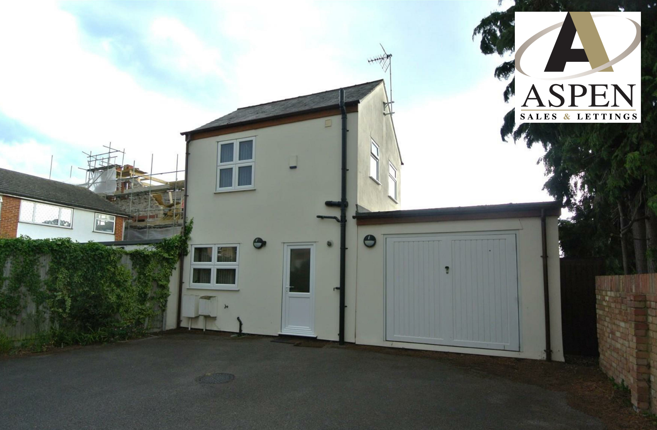
Coach House Chesterfield Road, Ashford, TW15 3PU
